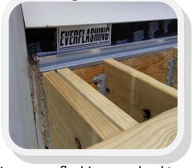
Improper flashing may lead to rot over time. Flashing should run from top to bottom between the house and the ledger. There should be counter flashing on the house that bends over the ledger and joists covered by house wrap.
