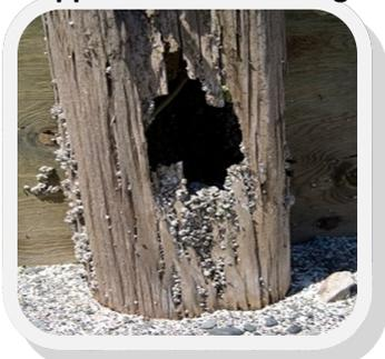
Investigate the deck support posts/pilings for bug damage, rot, or decay. Inspect rot with a screwdriver or ice pick. Decay may be present in wood if you can easily penetrate  $\frac{1}{4}$  –  $\frac{1}{2}$  inch, break off a sliver of wood without splinters, or if the wood is soft and spongy.
