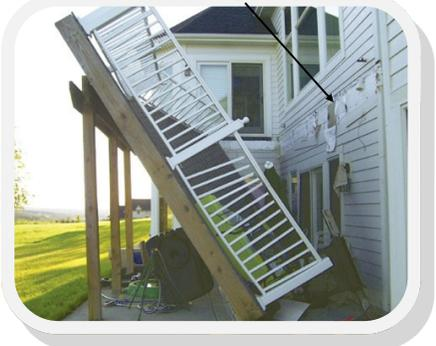
Closely check the attachment points between the deck and the house, including the ledger and fasteners. If the deck is connected to the house with a ledger, it should be attached with 5/8 inch bolts. Pay close attention to corroded fasteners.
