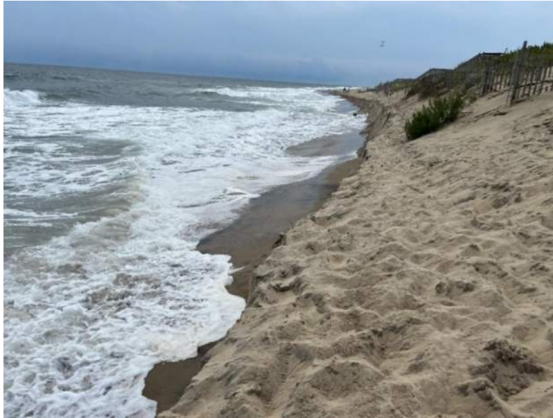
Figure 5-21. Scarping adjacent to McCall Ct. on July 27, 2024. (D. Ryan Photo)
