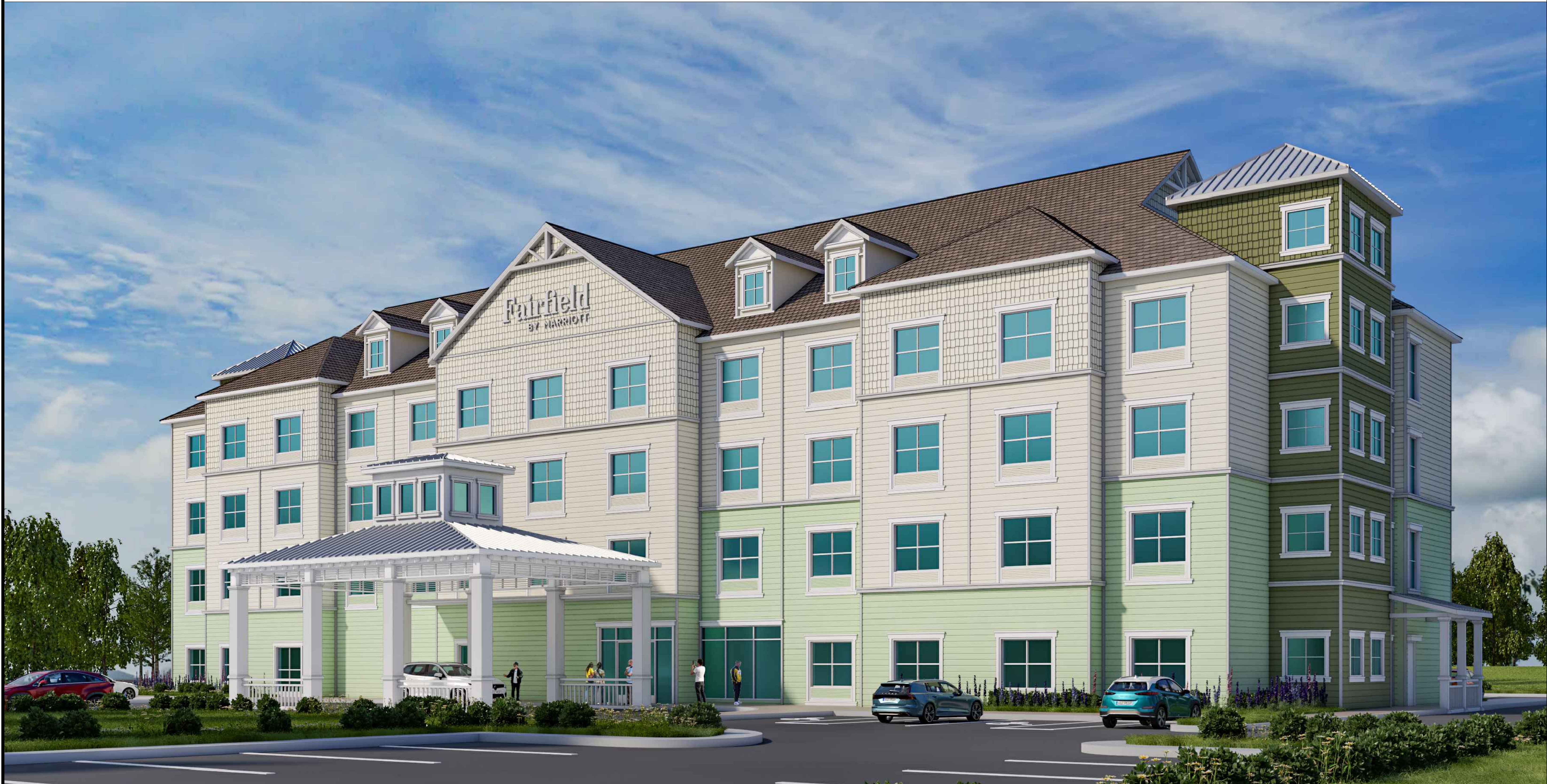
FRONT VIEW FROM NORTH-EAST CORNER
