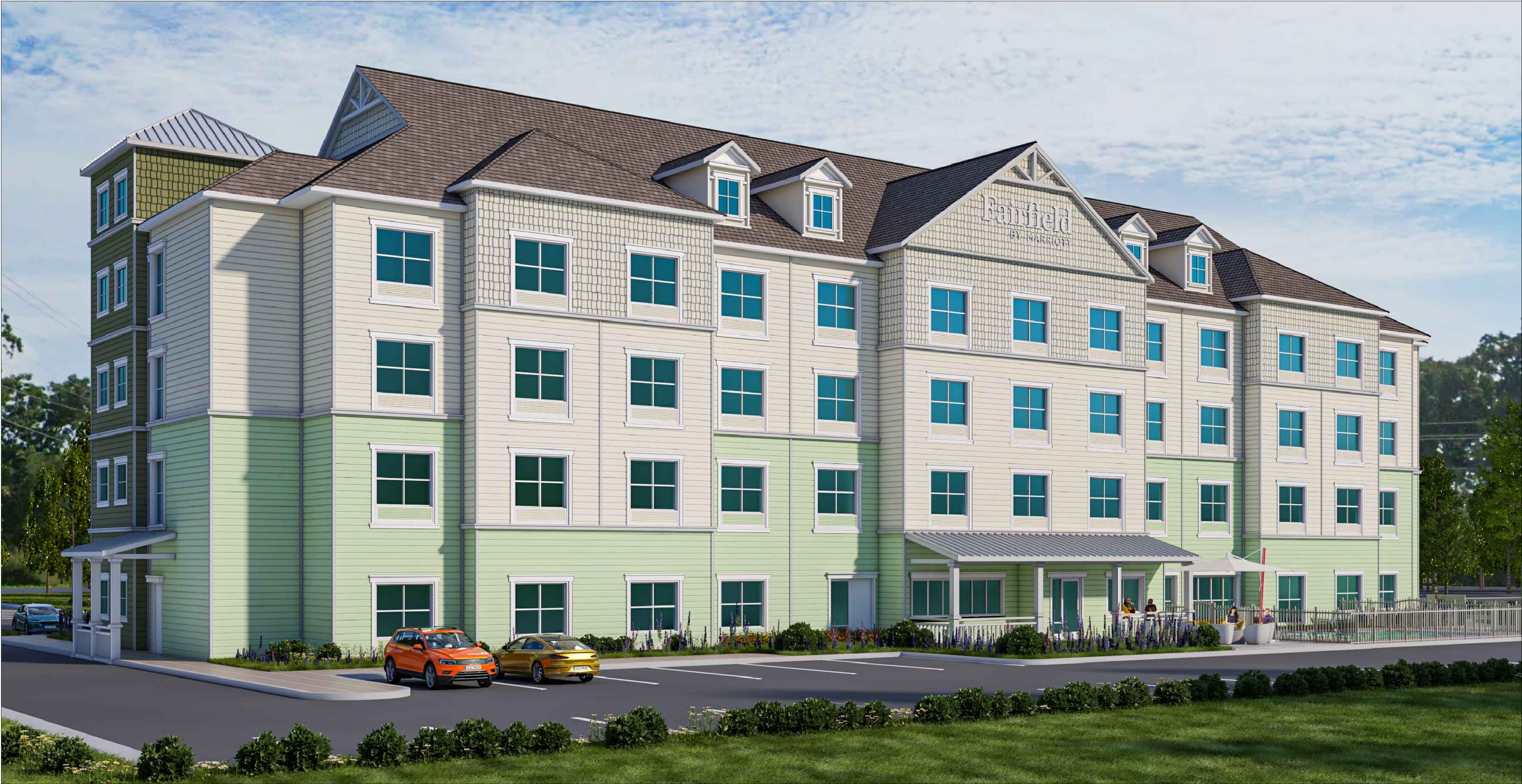
VIEW FROM NORTH-WEST CORNER
