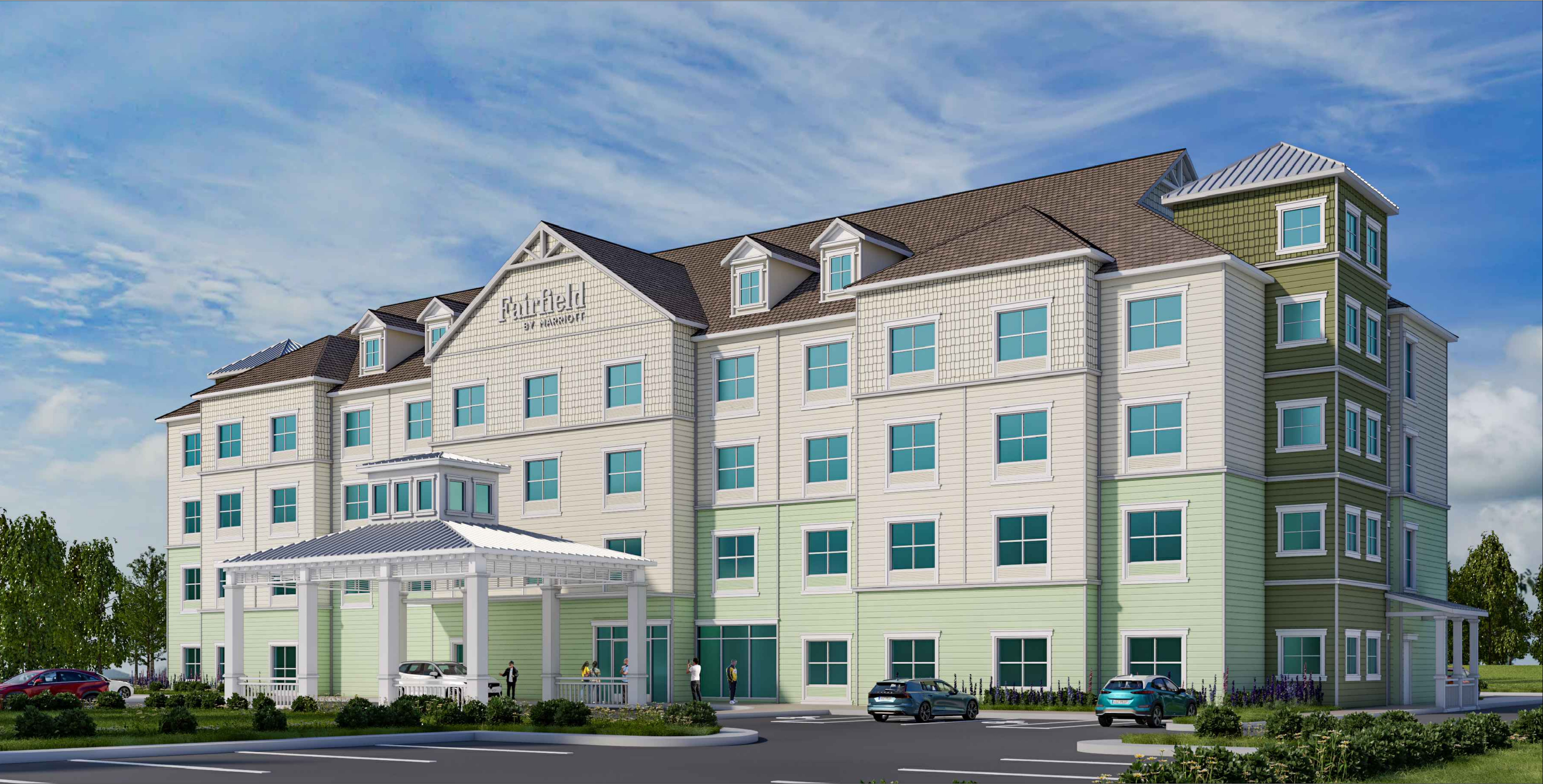
FRONT VIEW FROM NORTH-EAST CORNER
